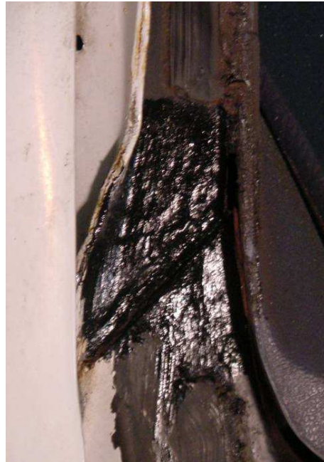
(Same area treated using treatment process)
