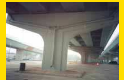
Case study provided by Vector Corrosion Technologies.
