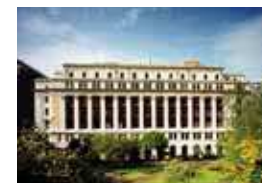
The Arkwright House, Manchester, United Kingdom was cathodically protected using Ebonex in 1998.
