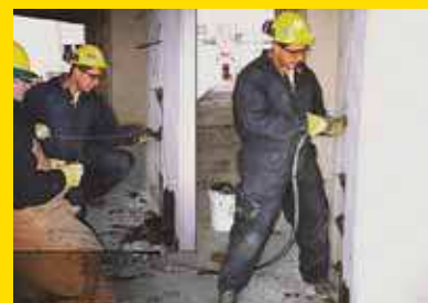
Case study provided by Vector Corrosion Technologies.
