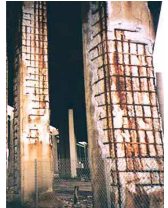
These bridge columns had to be demolished and rebuilt because the corrosion was too far advanced.
