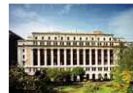
The Arkwright House, Manchester, United Kingdom was cathodically protected using Ebonex in 1998.
