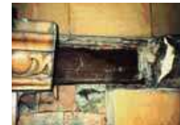
Example of steel beam corrosion causing failure of the decorative terra cotta facade.
