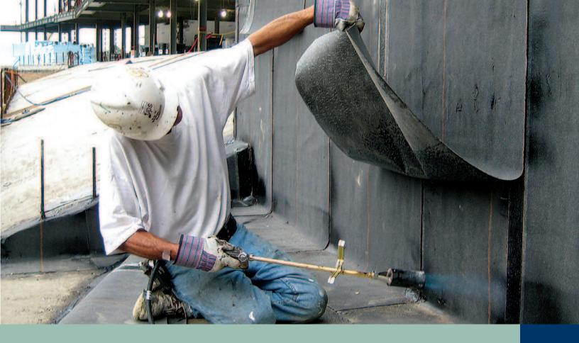
**HEAT APPLIED SOLUTIONS FOR WATERPROOFING FOUNDATIONS**
