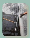
SopraSeal H Hot-applied, rubberized asphalt waterproofing membrane for plaza and parking decks
