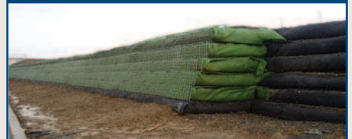
Wrapped Face Wall
