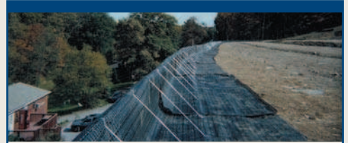
Wrapped Face Slopes
