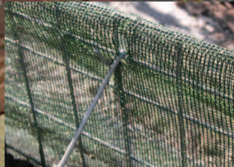
Miramesh® GR Biaxial reinforcement geosynthetic comprised of green polypropylene fibers.
