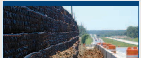
Temporary Retaining Wall
