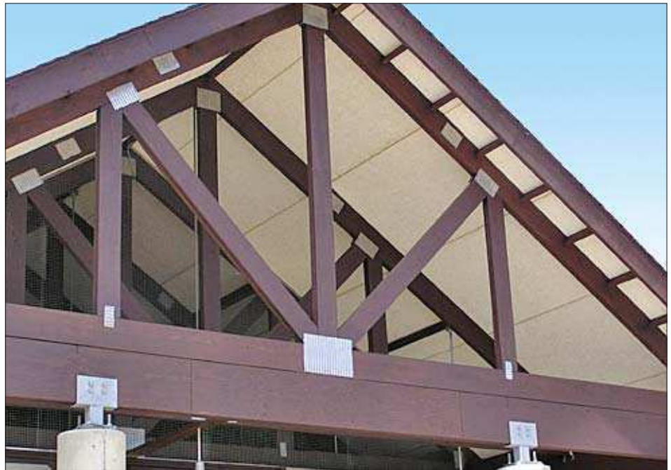
Pool House Roof Deck
