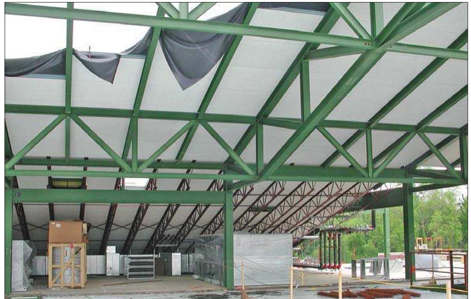
Swimming Pool Roof Deck
