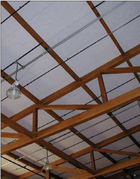
Tectum Roof Deck Over Wood Truss
