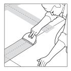
Fill joints with latex-fortified mortar or Type 1 organic adhesive and immediately embed Durock tilebacker tape or equivalent alkali-resistant, fiberglass mesh joint tape.
