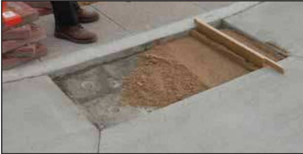
Step #3 - Sand Set Installation - Screed 1/4" masonry sand.
