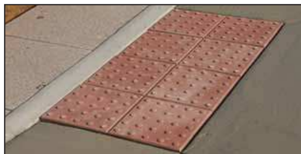
Step #1 - Wet Set Installation - While concrete is still wet, inbed pavers into cavity.
