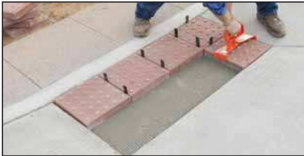
Step #3 - Thin Set Installation - Set pavers. Be sure pavers are fully set into thinset. (Back buttering may be necessary.)
