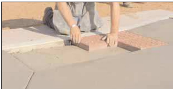
Step #1 - Wet Set Installation - While concrete is still wet, inbed pavers into cavity.
