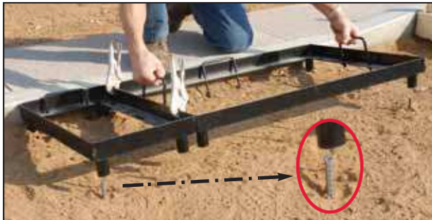
3- Set block-out frame so rebar sits inside the frame legs.
