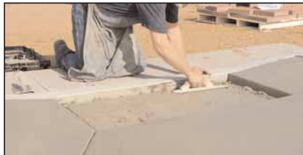
7- Pull out frame. Bull float area to receive ADA pavers.
