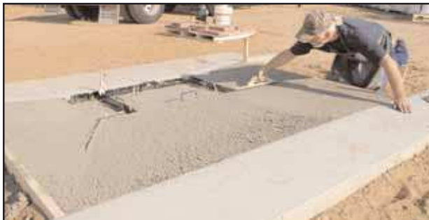
5- Pour concrete into and around framework. Level concrete and bull float area.
