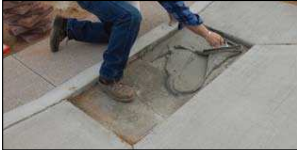
Step #1 - Thin Set Installation - Apply thin set with 1/4" x 3/8" notched trowel. Exterior grade.
