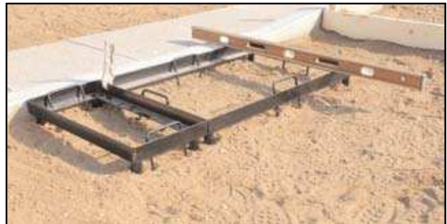
4- Set block-out frame to final grade by tapping on framework.
