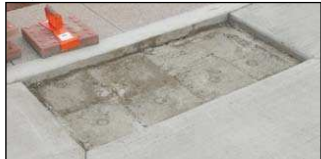
8- Allow concrete to cure. Use the following guidelines based on installation method. Note: If using wet set, do not allow concrete to cure.
