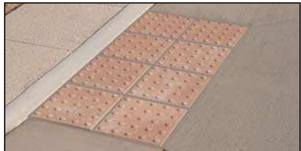
Step #4 - Thin Set Installation - Grout all joints with an exterior based grout. Complete.
