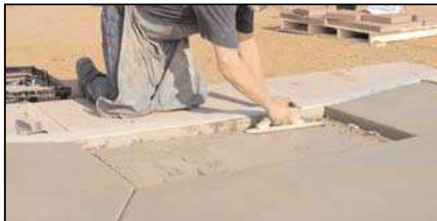
7- Pull out frame. Bull float area to receive ADA pavers.
