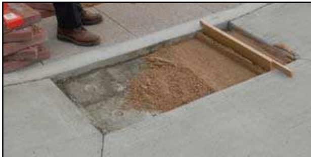
Step #3 - Sand Set Installation - Screed 1/4" masonry sand.
