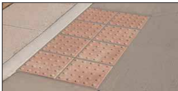
Step #4 - Thin Set Installation - Grout all joints with an exterior based grout. Complete.
