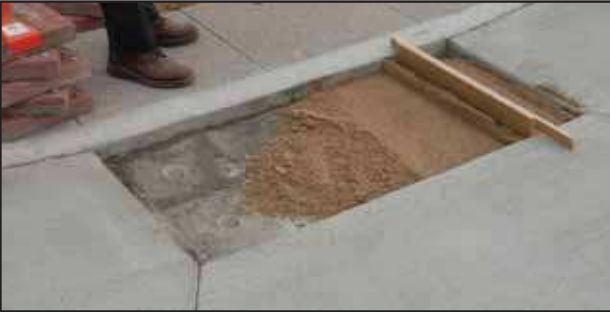
Step #3 - Sand Set Installation - Screed 1/4" masonry sand.
