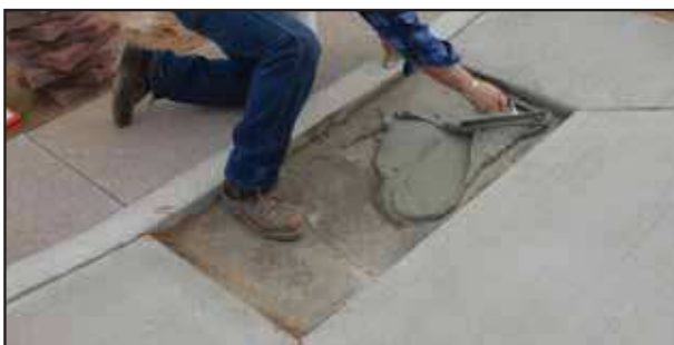
Step #1 - Thin Set Installation - Apply thin set with 1/4" x 3/8" notched trowel. Exterior grade.
