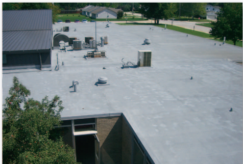
The R2R silicone coating is now ready to be applied to create a new, high performance silicone roof.
