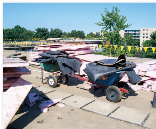
Old EPDM roofing material is removed.
