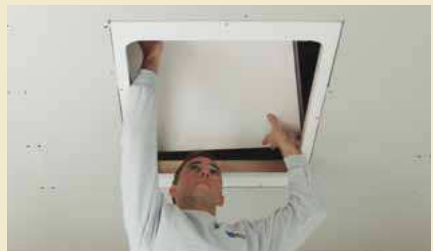
3. Install drywall and place access panel in opening.
