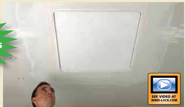
4. Tape and apply drywall compound.
