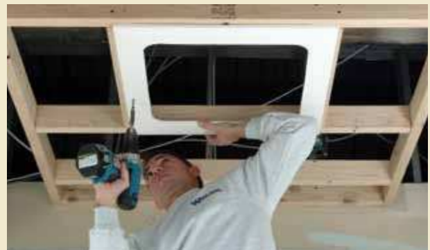
2. Mount Stealth surround with drywall screws.
