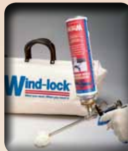
3 Shake can for 1 minute and purge air from gun.
