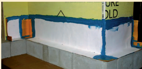
Specially designed nozzle creates proper geometry for liquid termination bar
