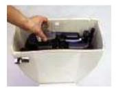
Step h. Turn on the water supply and check all lines carefully for leaks. To insure that the FVC o-ring is properly seated, pour water onto the top of the FVC and check for air leaks. Test flush the unit several times to clear excess air and continue use.
