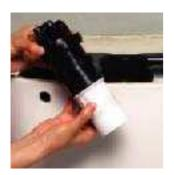
Step 7. Inspect the FVC large o-ring at the top of cartridge and also check the lower o-ring for damage or if it is properly seated. NEVER USE ANY LUBRICANTS ON ANY OF THE PARTS OF THE ECOFLUSH AS THIS WILL VOID THE WARRANTY AND CAUSE DAMAGE TO THE PARTS.
