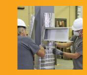
Installing multiple layers of 3M<sup>™</sup> Interam<sup>™</sup> Endothermic Mat E-5A-4 flexible wrap allows you to tailor the desired amount of fire protection—up to 4 hours for structural steel.
