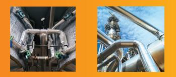
When 3M<sup>™</sup> Interam<sup>™</sup> Endothermic Mat E-5A-4 is applied to vessel skirts and pipelines, it minimizes the effects of fire exposure by flame impingement in order to reduce the steel's rate of temperature rise and to delay structural failure.
