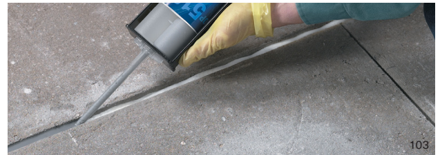
Make fast work of lengthy expansion or control joints and other larger jobs with the heavy-duty manual applicator and 12 fl oz. duo-pak cartridges.
