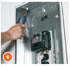
The bottom or top of the steel box may be penetrated by up to 2" metallic conduit. See system parameters.
