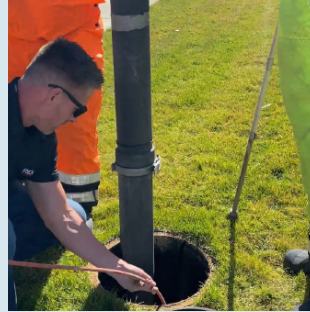
Vacuum removal of debris
