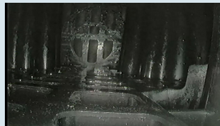
Camera view of clean tank
