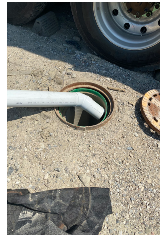
4" pipe with 45 ° elbow to guide push camera
