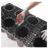
Modules can be easily cut in half to allow integration into the overall system.
