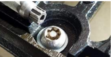
Tamper-resistant bolts for 4-Bolt grate require tamper-resistant drive bit
