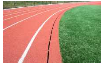
Drainage Slot 0.5" ADA compliant drainage slot offset from the center of the channel
