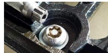
Tamper-resistant bolts for 4-Bolt grate require tamper-resistant drive bit
