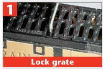
To close, place hook part of tool into 'V' and push towards rail.
