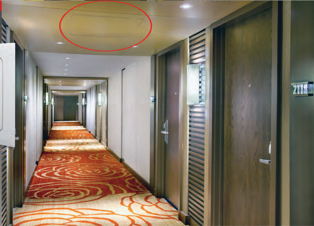
Glass Fiber Reinforced Gypsum, GFRG-R Glass fiber reinforced gypsum, ceiling access doors are designed to blend seamlessly into drywall ceilings
