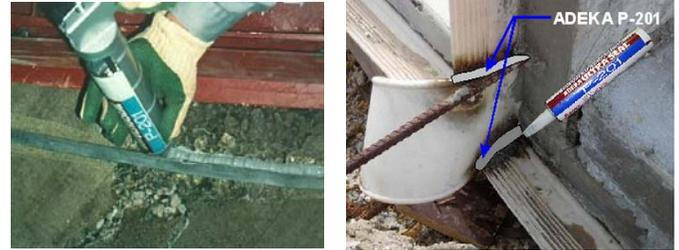
Use to fill rough areas when using Adeka strip products. Apply on PVC waterstop weld seams.
