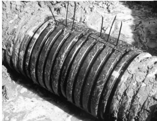
Figure 3 Split Band Installation
