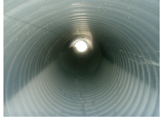
Smooth Interior Wall
