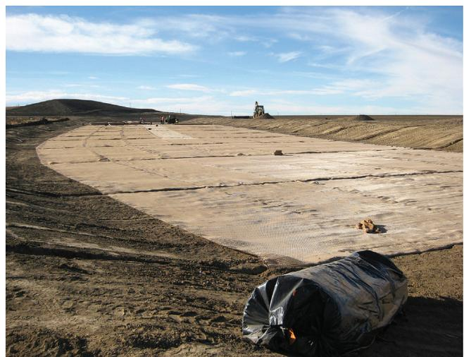
**High-performance turf reinforcement mat with ultra-violet resistance for up to a 50-year design life in semi-arid conditions.**
