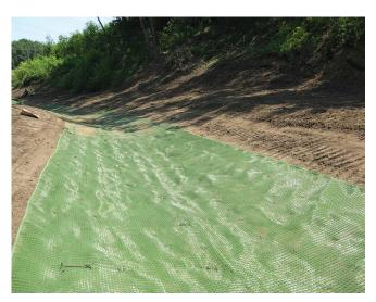
Woven turn reinforcement mat used for steep slope channel stabilization.
