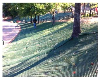
Slope stabilization utilizing an armor system.
