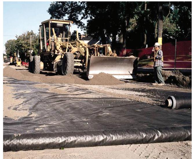
**A woven geotextile is placed on a roadway prior to paving. An ADS woven geotextile allows aggregate layers to maintain their original design thickness.**
