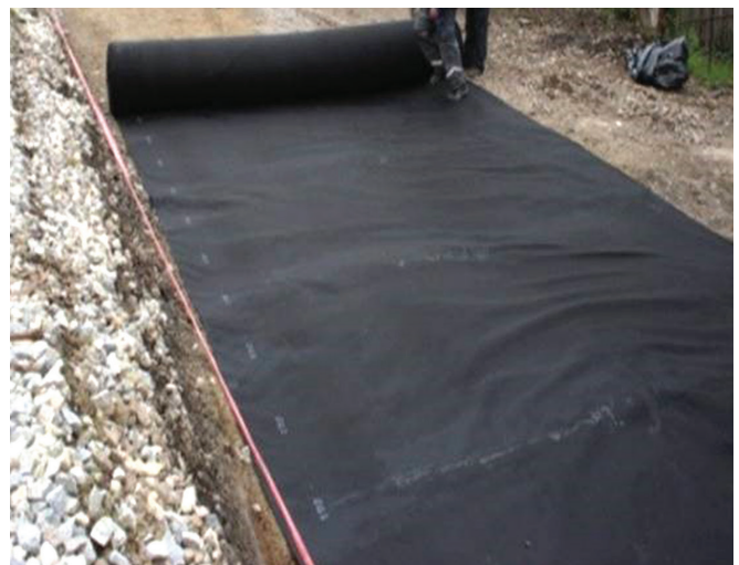
Robust nonwovens stabilize subgrades and extend road life.
