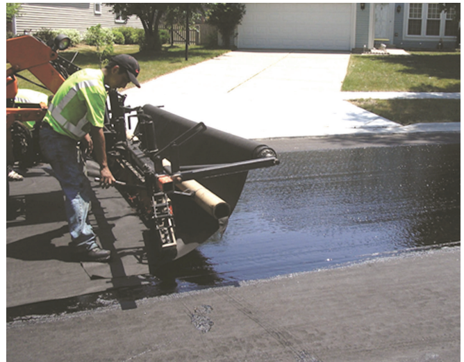
Paving fabric provides additional support to asphalt layers on roadways.
