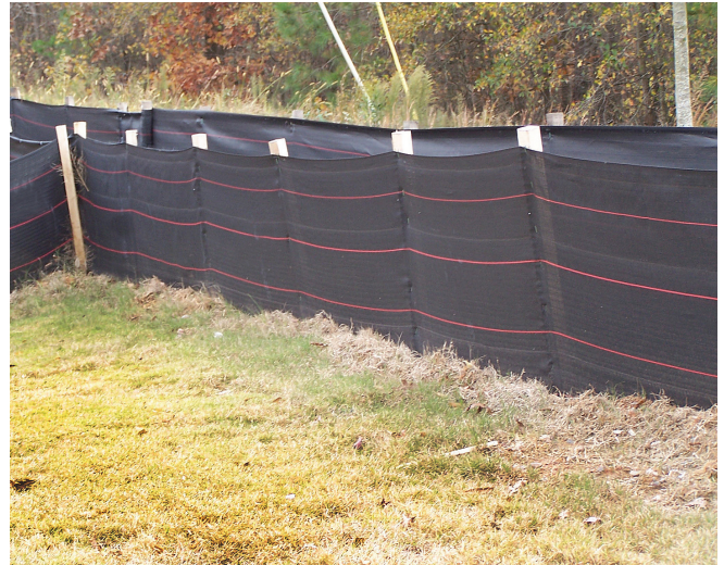
Silt fences trap sediment before it can pollute surface waterways.
