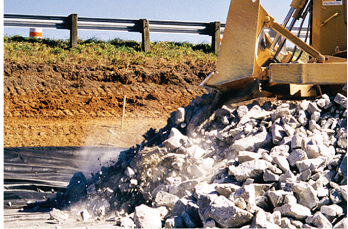
ADS nonwoven geotextiles act as a filter to relieve hydrostatic pressure and prevent soil migration beneath hard armor, such as rock riprap.
