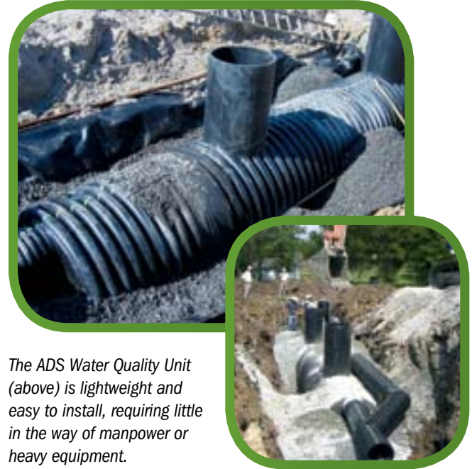
A bypass system (above right) is installed to prevent water flows greater than the first flush from re-suspending captured pollutant particles.
