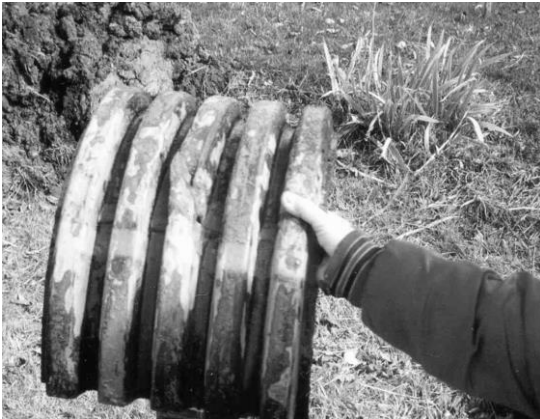
Figure 2 Pipe Cut Location
