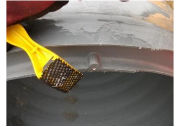
Figure 10: Finishing the Weld
