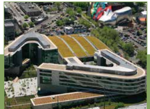
Gates Foundation Garage - Seattle, WA
