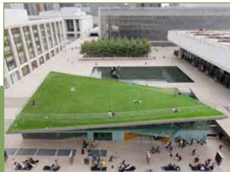
Hypar Pavilion at Lincoln Center - New York, NY
