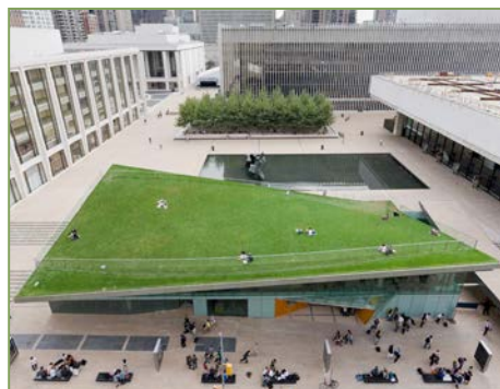
Hypan Pavilion at Lincoln Center - New York, NY
