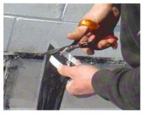
Cut off one corner of the plastic bag to make a spout and then squeeze the contents out of the bag in the desired area. Trowel the material to the desired thickness.
