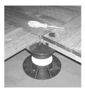
Insert FS1 washer in the slot between the top slat and bottom brace.
