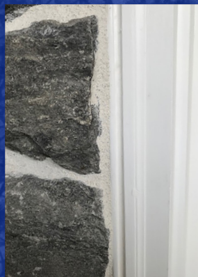
E-Z Bead Allows for a Smooth, Thin Caulk Joint
