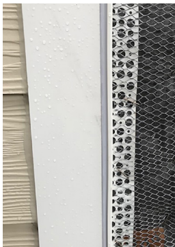
Bond Breaker Tape Releases from the Flexible Strip After Caulking to Prevent Cracking & Joint Failure
