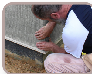
Installation of Lath
