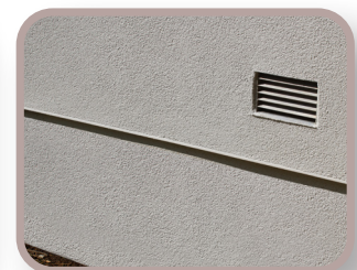
Drain Screed on Finished Wall
