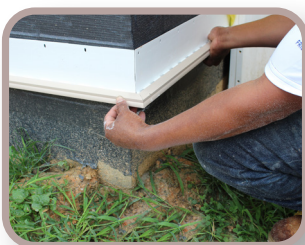
Installation of Drain Screed
