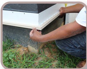
Installation of Drain Screed
