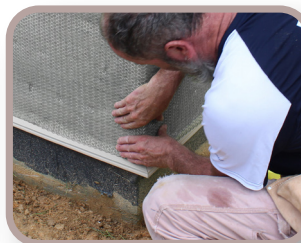
Installation of Lath
