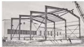
1965 Plant Expansion in Birmingham, AL
