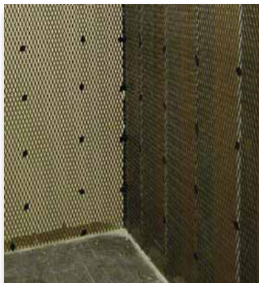
Security Mesh™ Behind the Drywall Penetration Barrier
