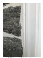
E-Z Bead Allows for a Smooth, Thin Caulk Joint
