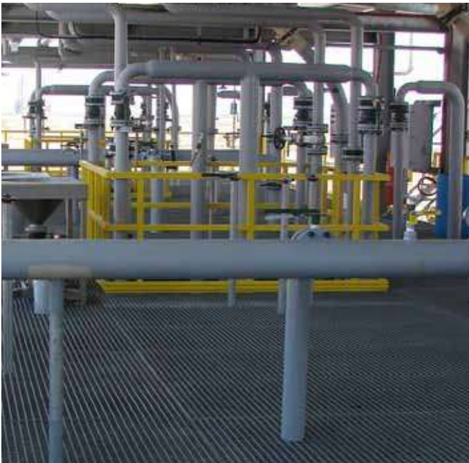
Custom FRP Grating & Handrails
