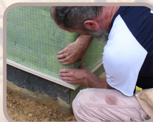
Installation of Lath
