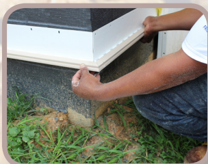
Installation of Drain Screed
