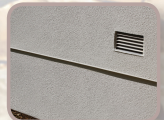
Drain Screed on Finished Wall
