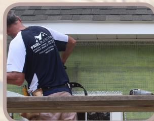
Installation of E-Z Vent
