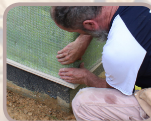
Installation of Lath
