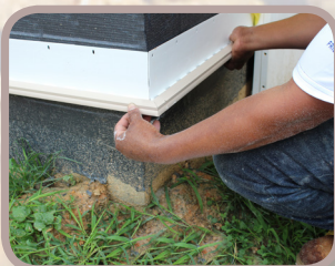
Installation of Drain Screed
