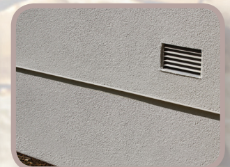
Drain Screed on Finished Wall
