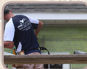
Installation of E-Z Vent
