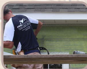
Installation of E-Z Vent
